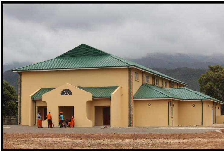
Moshate Community Hall
